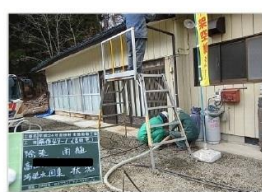
High pressure water cleaning of a drain pipe
