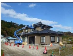
Wiping off rooftop and walls
