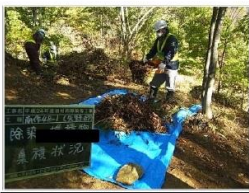
Mowing and removal of sludge
