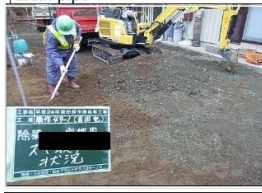
Removal of crushed stones and topsoil, and cover with clean soil
