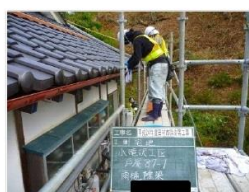
Wiping off a gutter
